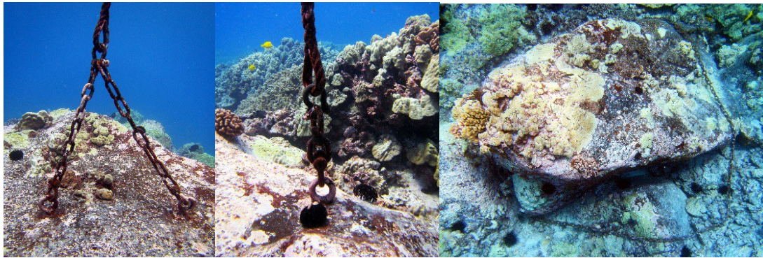
Figure 11. Day-use moorings at Keauhou Bay: ( left ) middle south with double pin anchor, ( middle ) inside north with single pin anchor, and ( right ) south chain which is only loosely wrapped around a boulder.
